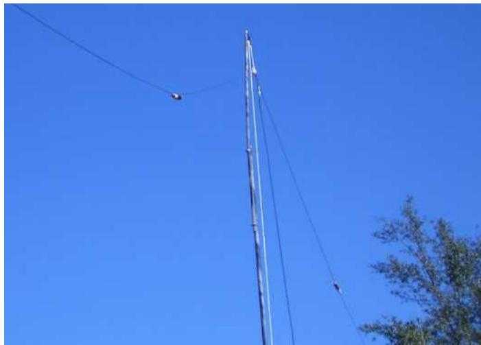
Center Support Mast – 25 feet
