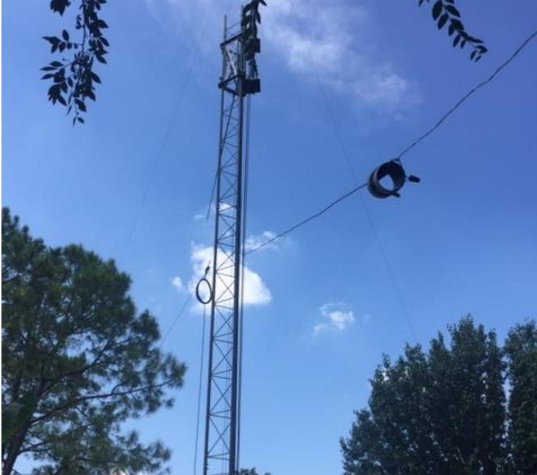
Using my MFJ 269B Antenna Analyzer, I found that it had to be adjusted as it was too low in frequency (too long) as built. Using the uninsulated aluminum end sections, which made it easy to just fold back on itself, I shortened one side a few feet and found a sweet spot at 3910. SWR was about 1.7:1 at the end of the 70 feet of RG58. Not going to get any better than that at 20 feet. SWR will get lower as the antenna is moved higher and the feed Z increases toward 50 ohms.
